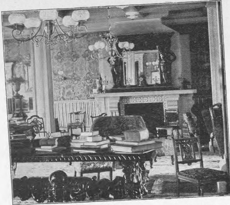
No. 133.—A CHIMNEY AND MANTEL-PIECE OF CONCRETE IN THE DRAWING-ROOM OF THE HOTEL CASA-MONICA, ST. AUGUSTINE.
