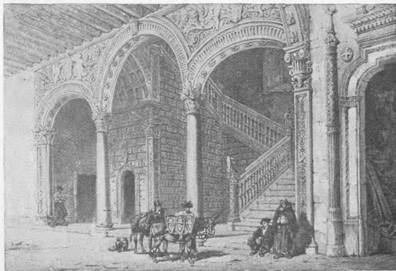
No 56.—STAIRCASE, TOLEDO. SPANISH COURT. R.
